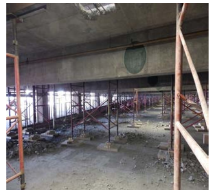
Structural Garage Improvements
