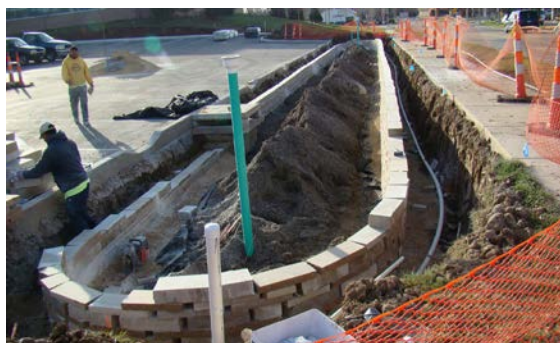
Government Center Parking Lot Expansion
