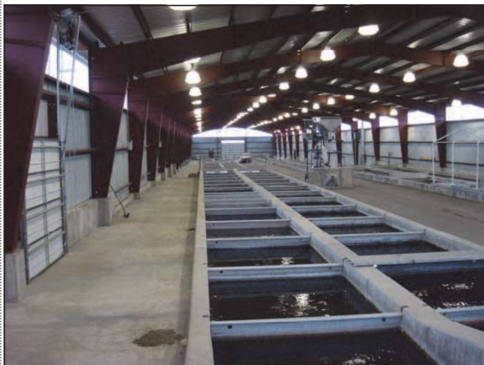
Covered raceways at the Whiterocks State Fish Hatchery
