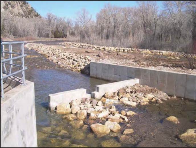
Reconstructed Tabby Diversion on the Duchesne River
