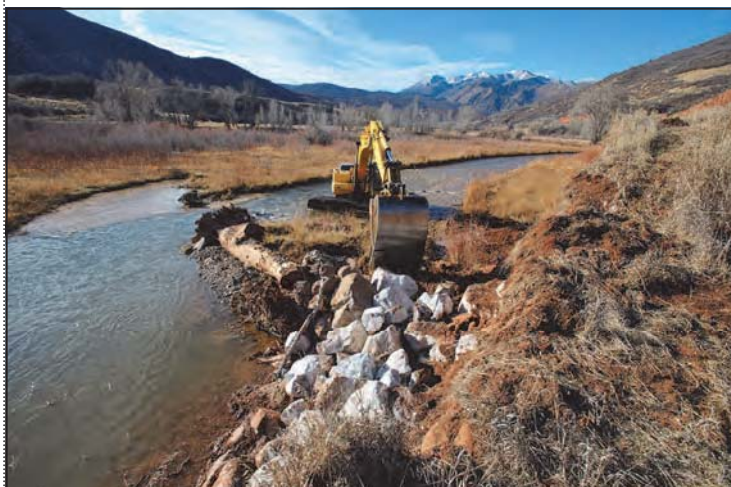
Installation of log and rock barb in main Diamond Fork channel
