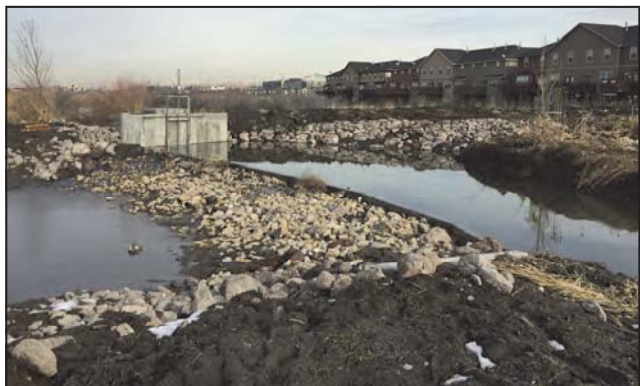
A new diversion structure (shown left) installed in 2015 by the Mitigation Commission and Bureau of Reclamation, provides adequate flows to support the restored Willow Creek wetland complex (shown right), while ensuring high flows are delivered to the Jordan River, and water rights are met.
