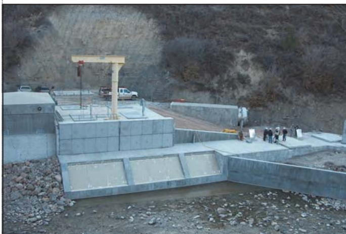
Sixth Water Flow Control Structure
