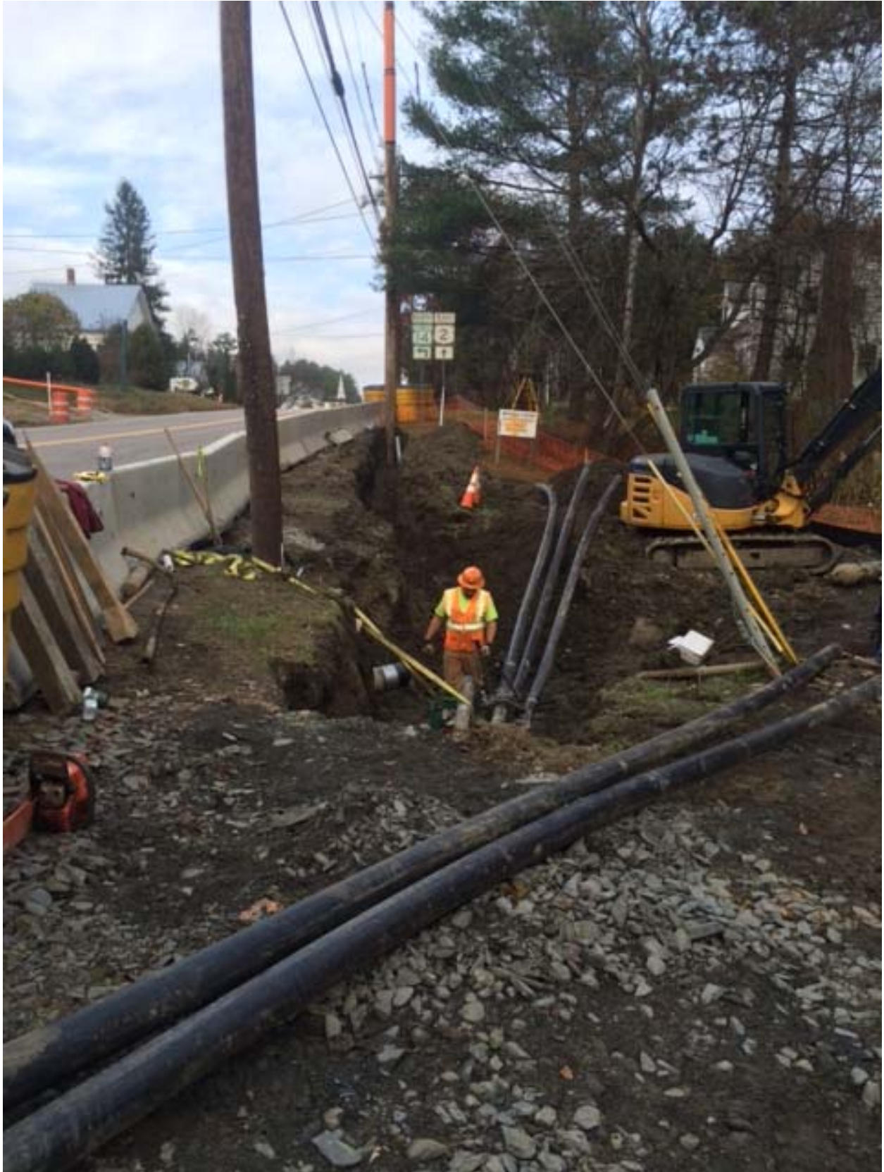
Installation of telecommunications conduits (five 4-inch pipes) is nearly completed.
