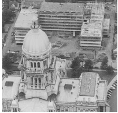
Construction of the Stratton building, west of the Capitol, began in 1954.
