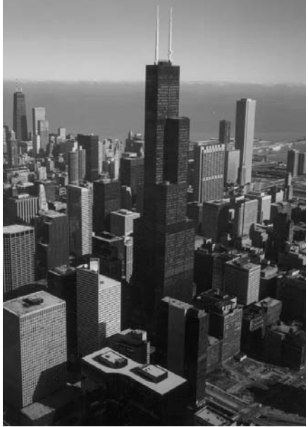
At 1,454 feet, the Sears tower was the tallest building in the world until February 1996.
