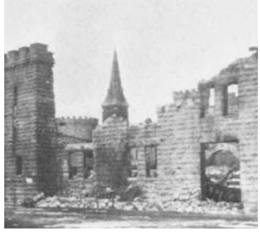
The State Arsenal in Springfield after being destroyed by fire in 1934.
