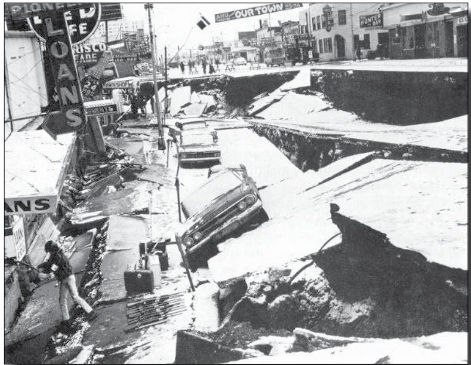
Anchorage 4th Avenue slide (USGS photo library)
