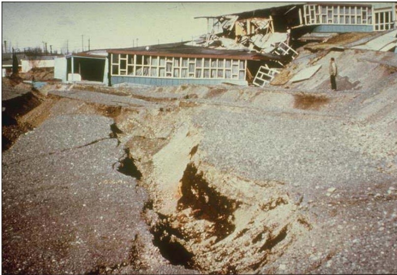
Figure 1. Destruction of Government Hill School in Anchorage as a result of landsliding triggered by the 1964 earthquake.
