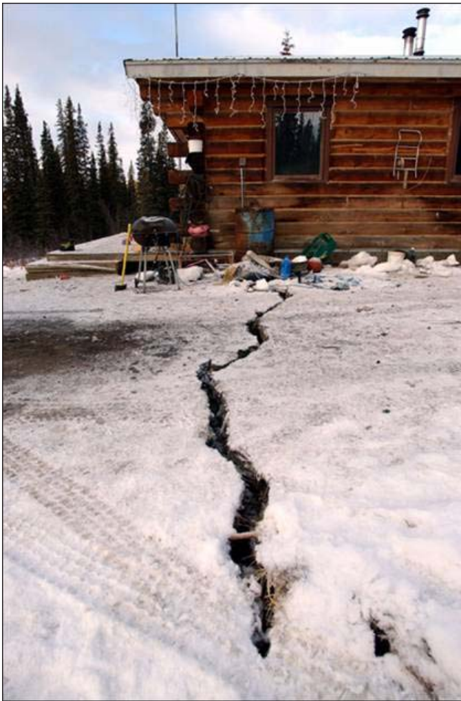
Figure 4. Ground cracking in Mentasta as a result of the 2002 magnitude 7.9 Denali fault earthquake.
