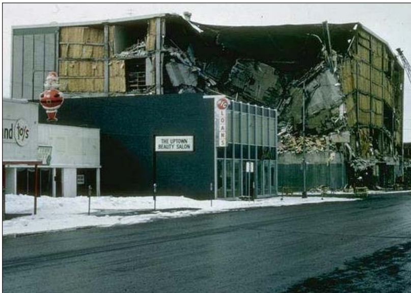
Figure 2. Collapse of the J.C. Penney building in Anchorage as a result of strong ground shaking during the 1964 earthquake.
