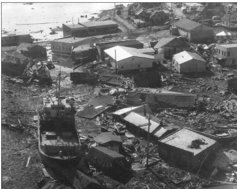
Figure 3. Tsunami damage in Kodiak resulting from the 1964 earthquake.
