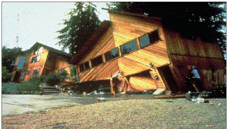
Figure 5. Shaking damage to residential facilities from the 1989 Loma Prieta, California, earthquake.
