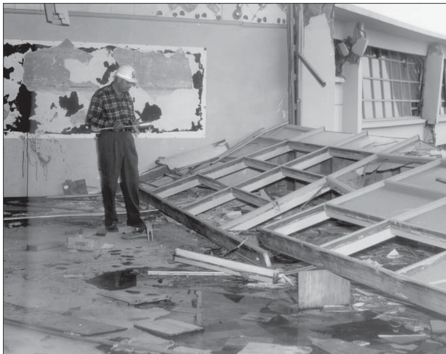
Figure 4. Anchorage High School, 1964 Alaska earthquake (photo credit Anchorage Museum).
