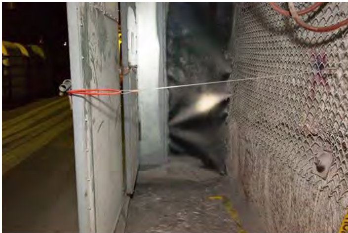
Air Lock Doors Wired Open
