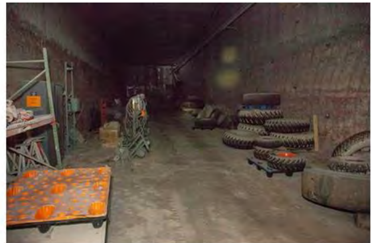
Combustible Loading in the Mine
