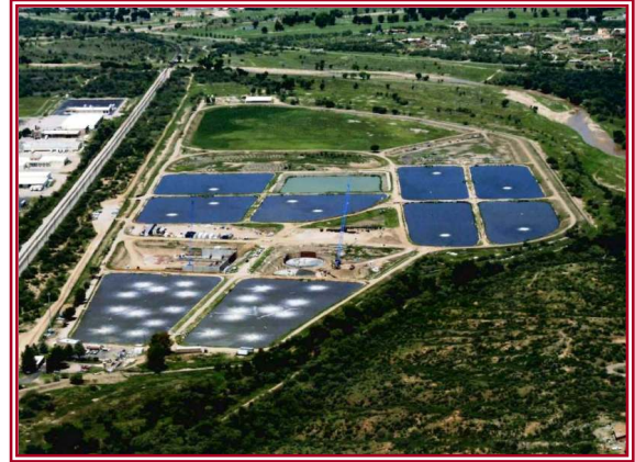
Nogales Int'l Wastewater Treatment Plant
