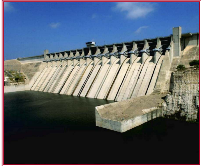
Amistad Storage Dam
