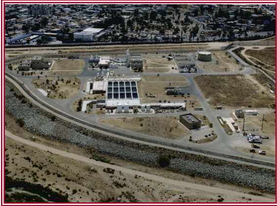
South Bay Int'l Wastewater Treatment Plant
