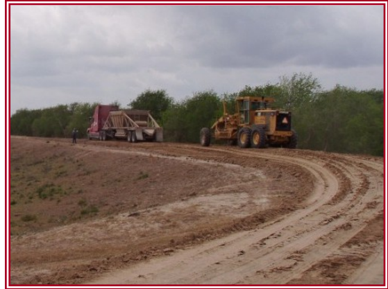
Lower Rio Grande Levee Improvements
