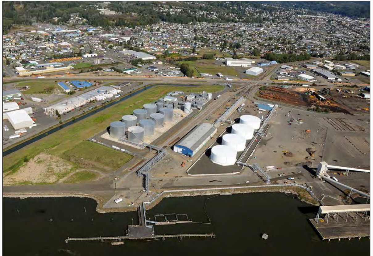
The Contanda storage tanks at the Port of Grays Harbor. In addition to the four white tanks that hold 320,000 barrels, five much larger tanks would be built to the right of these in this project. Currently, methanol and magnesium oxide are stored there. Photo by Larry Workman
