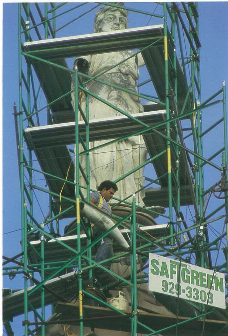
Above: Intricate scaffolding permitted extensive close-up evaluation of the statue's condition.
