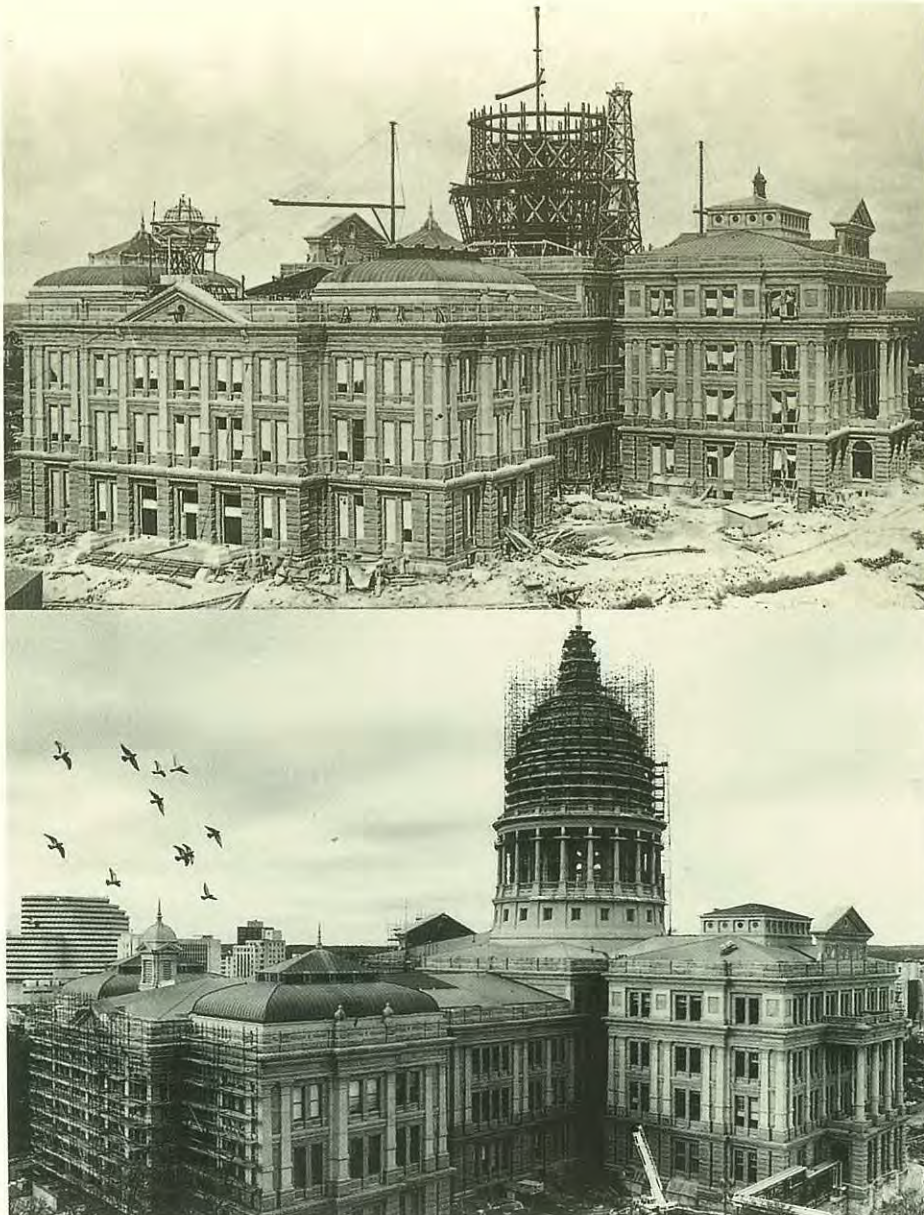
Capitol Construction 1880's and 1990's
