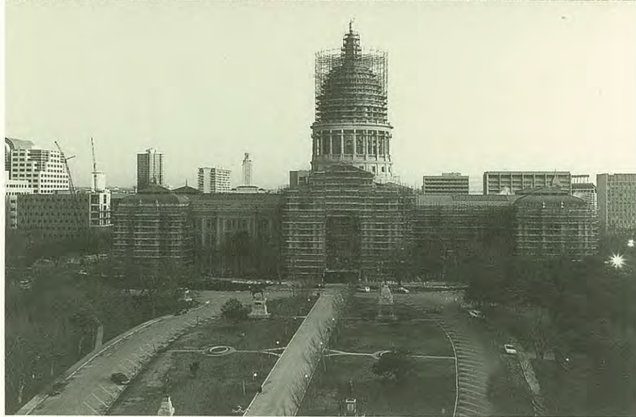
Capitol Construction 1880's and 1990's
