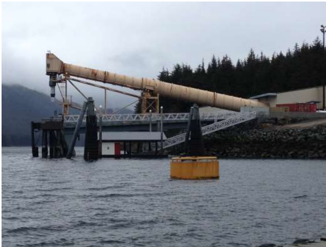
Figure 6-1. Ore loading dock at the HGCMC
