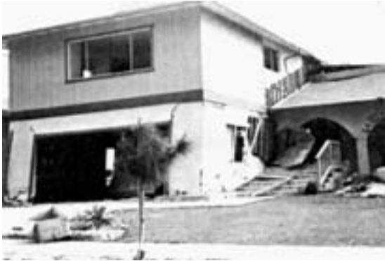
Figure 1 - San Fernando Earthquake, Feb. 9, 1971 Severely damaged split level one- and two-story wood frame dwelling. The one-story portion dropped about 3 feet.
