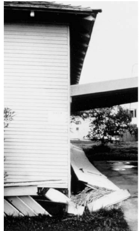
Figure 12 - Damage to home due to crawl space wall failure.
