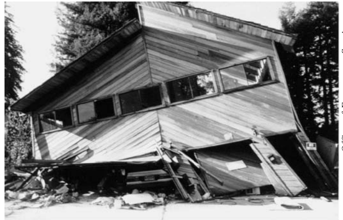
Figure 25 - This mountain home was built over a garage, and its walls were not strong enough to withstand an earthquake.
