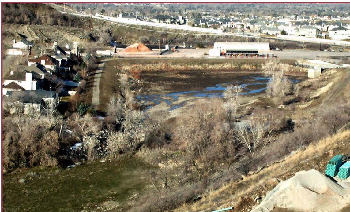
Figure 26, Debris Basin at the Mouth of Big Cottonwood Canyon
