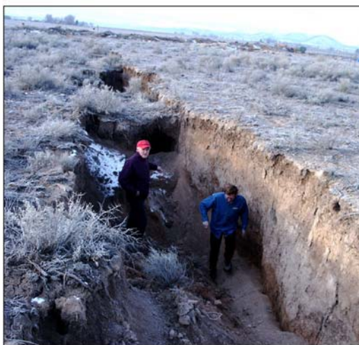
Figure 16, Beryl-Enterprise Area Ground Subsidence and Cracking Source: Utah Geological Survey, 2005
