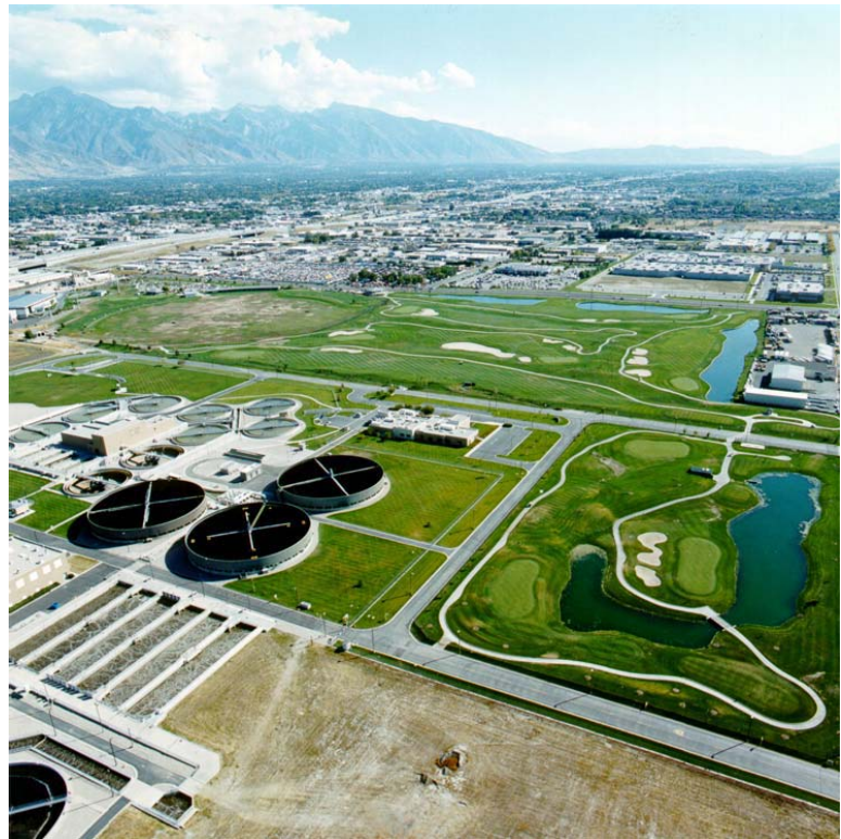
The Central Valley Golf Course receives approximately 0.6 million gallons per day of reclaimed water from the Central Valley Water Reclamation Facility to irrigate its greens and fill the various decorative ponds. (Photo courtesy of Central Valley Water Reclamation Facility.)
