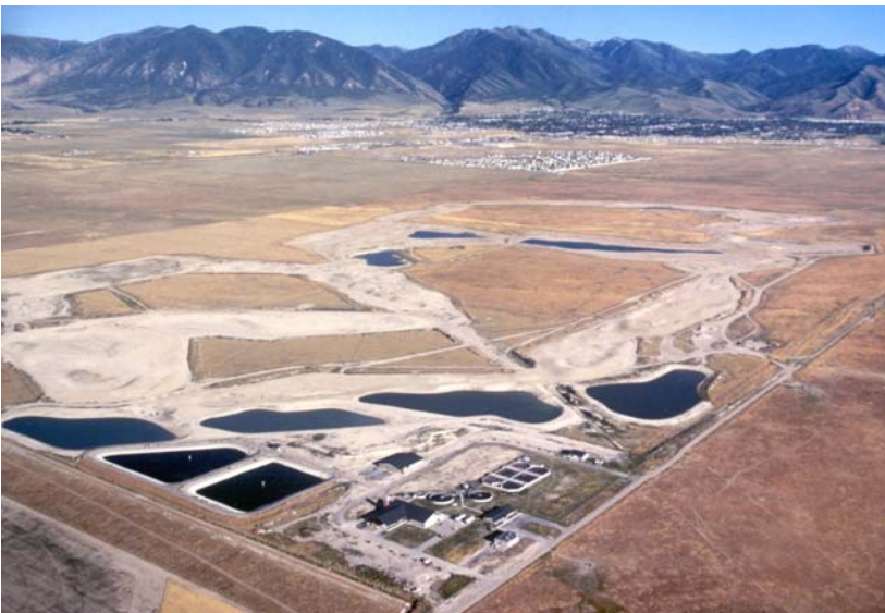
Aerial view of Tooele's Wastewater Treatment Plant and the golf course's lakes that store the reclaimed water for irrigation. (Photo courtesy of Tooele Wastewater Treatment Plant.)
