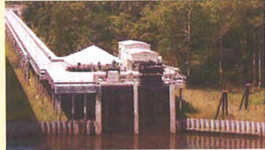
Ouachita River Alternative Water Supply Project intake structure in Union County near El Dorado - Photo courtesy of Union County Water Conservation Board
