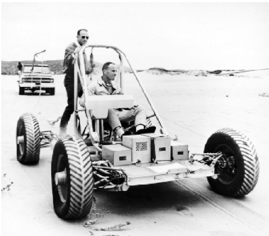
Astronauts Jack Lousma (seated) and Gerald Carr test the lunar roving vehicle mobility test unit on the sands near Pismo Beach, California.
