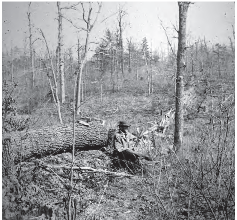
Federal entrenchments across Orange Turnpike about one mile west of Chancellorsville
