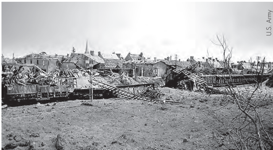
Destroyed railway in Carentan, c. June 1944
